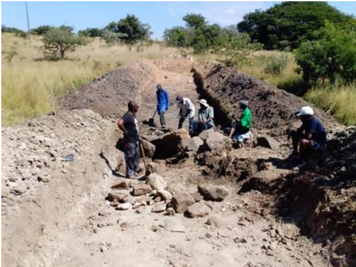
Plate 2: Villagers digging the weir foundation.
