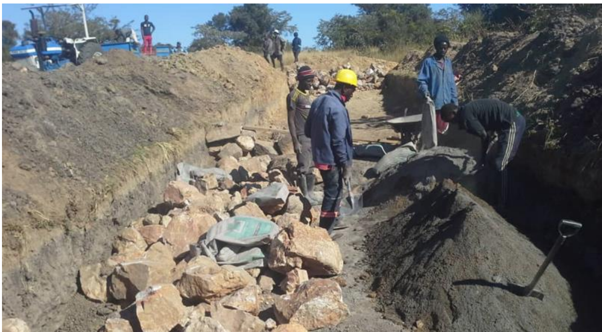
Plate 4: Weir Dam construction in progress
